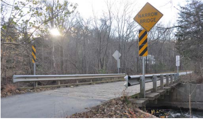
Route 638 bridge over South River
